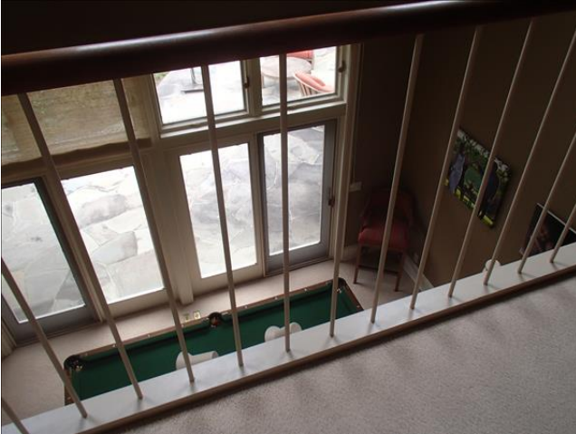
Living Room / Main Hall Interior Stairway(s) Attention
